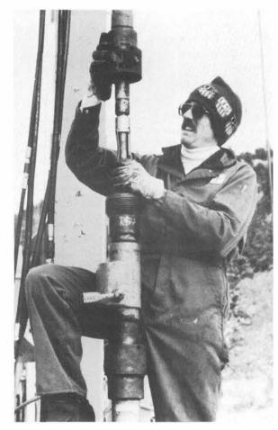
HOW HOT? — Joe Coquat of Geothermal Technology Division 4736 inserts a prototype of a high-termpature well logging tool into a Union Oil geothermal wellhead. Instrument passed first field test, operating at temperature of 275°C.
